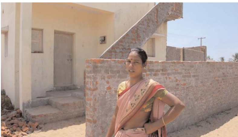
Raji stands in front of her new house, one of 101 built by an Oxfam partner in the village of Chettinagaram in the Indian state of Tamil Nadu. An Oxfam shelter evaluation revealed problems with the quality of the construction, as well as problems between the partner and the community. As there had been a delay in the construction, Raji invested her own savings to build the staircase. Oxfam reimbursed the costs and carried out the repairs outlined in the evaluation. (Photo: Marie Banu Jawahar/Oxfam)
