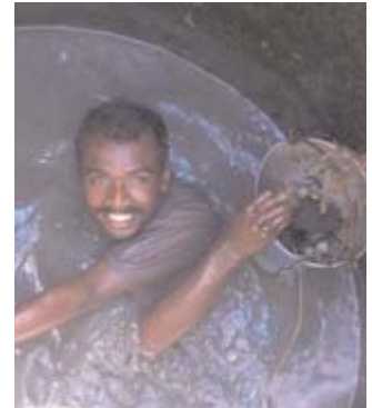
N. Kairuniananaitheven, a fisherman who lost his boat and nets in the tsunami, volunteered to clean the debris from the bottom of a well in Kathirawell, north of Batticaloa. Oxfam technicians had pumped saltwater from the well and it had refilled with groundwater. (Photo: Howard Davies/Oxfam)
